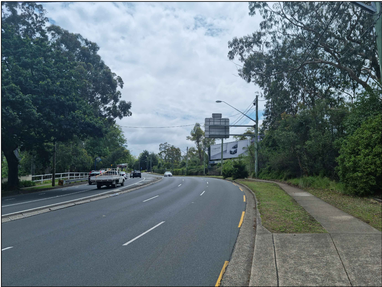
VIEW TOWARDS N - W
